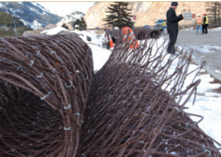
Coiled wire mesh sections rests on the side of I-70 awaiting helicopter hoist to construction side on Georgetown Hill. Georgetown Hill photos by John Gross, CDOT
