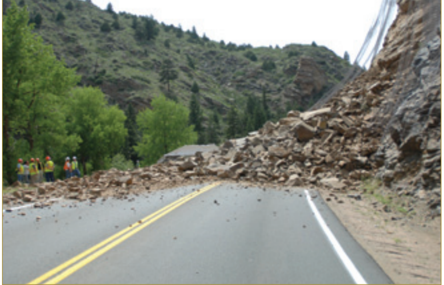
View of rocks on road. Note that wire stabilizing mesh installed last year still hangs from its top anchors.
