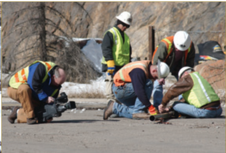
Crews prepare the metal spreader beam that will be attached to the wire mesh top to keep it from crumpling during transport.
