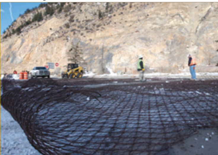
The mesh resembles a large chain link fence with sections 15 feet wide by 30 feet long and weighing 1,200 pounds.
